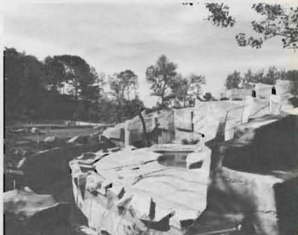
No more bars or cages to obstruct visitors' view of the bears, the moated grottos are the newest "look" at the Cleveland Zoo. Photo Courtesy of Schafer, Flynn, Van Dijk, Dalton, Grimm, Johnson Architects.
