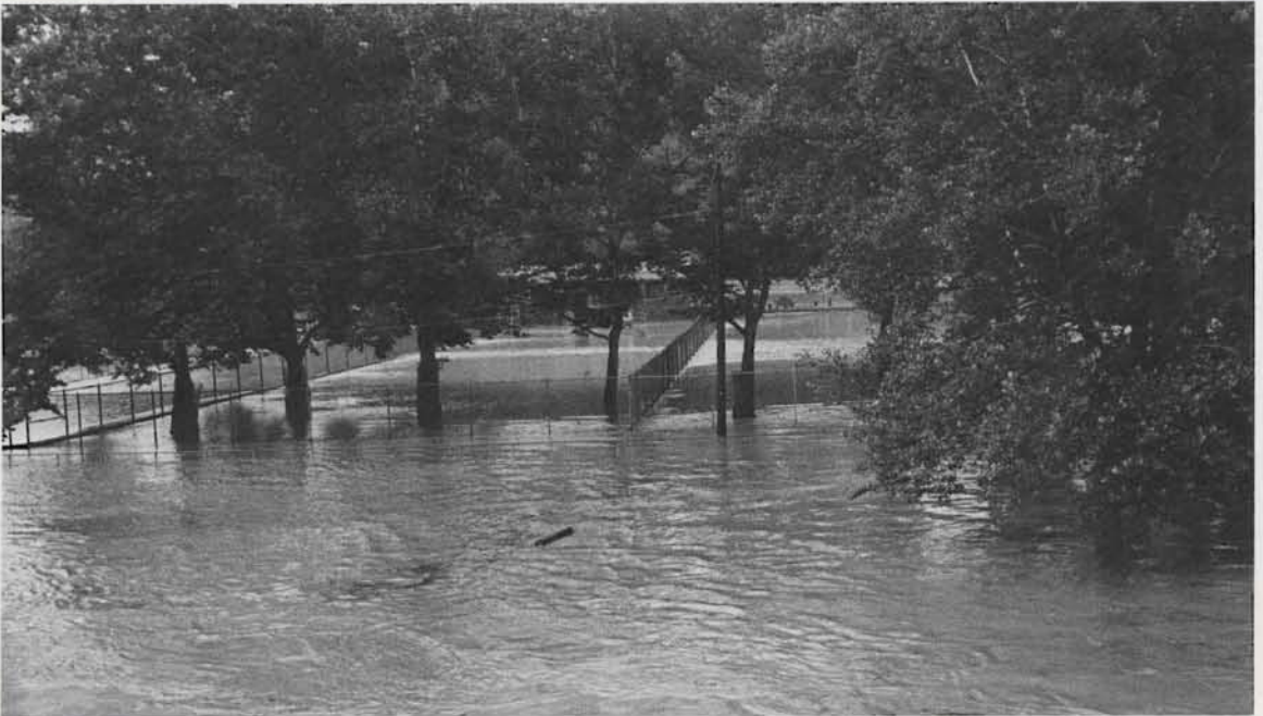
Flooding of Big Creek, which has plagued the zoo for many decades, will be eliminated when the U.S. Army Corps of Engineers re-channels the creek bed which currently follows a course through the main part of the zoo. The flood of 1964, pictured above, caused many thousands of dollars worth of damage. The flood control program, scheduled to begin in 1979, is to be completed in 1981.
