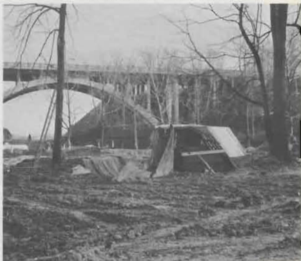
Hooved animal moat wall is protected from cold weather by canopy. Walls are of gunite construction (sprayed concrete over an expanded metal framework). Fulton Road Bridge and Goat Hill may be seen in center background.
